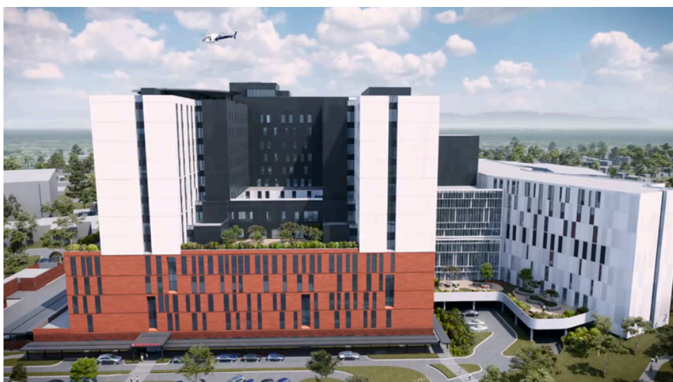
Figure 8. Nepean Hospital Redevelopment – Stage 1 and 2
